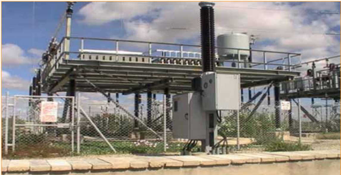
Figure 10: Dodoma Substation - Capacitor Banks
