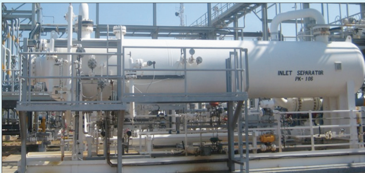
Figure: 11 The Production Separator at Songo Songo Gas Plant
